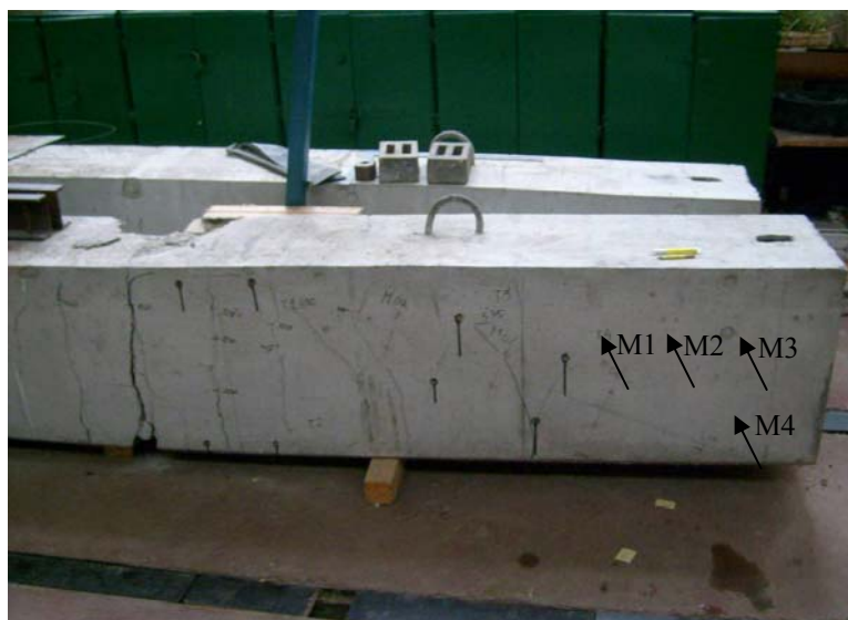
Fig 5. Tested beams in a longitudinal direction
